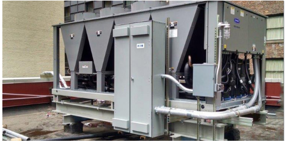
Donnelly installed a new air-cooled chiller system, allowing for less equipment, more efficiency, and better serviceability.
